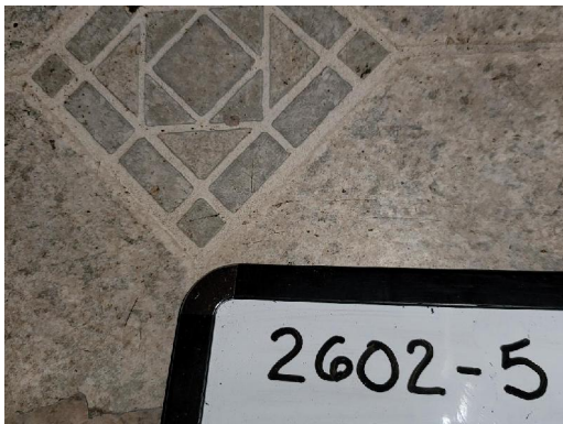
2602-5 12"x12" Floor Tile/Adhesive Interior Kitchen (Bottom Layer)
