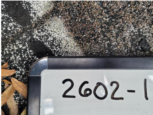
2602-1 Asphalt Shingle/Tar Typical Exterior Roof
