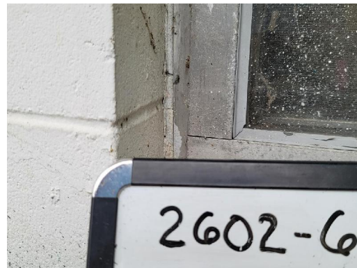
2602-6 Caulk/Off-White (3% Chrysotile) Typical Exterior Windows
